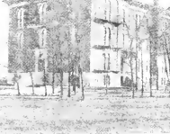
A view of the original college building built in 1869.
